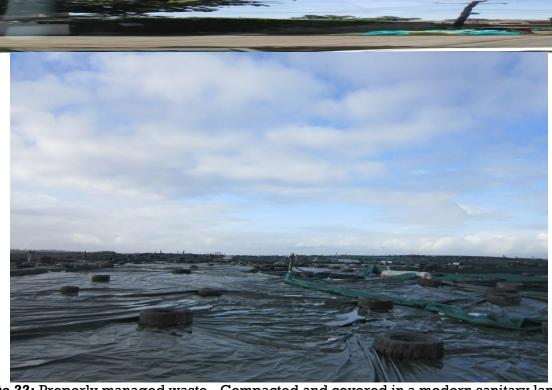
Plate 22: Properly managed waste - Compacted and covered in a modern sanitary landfill, Dublin.
